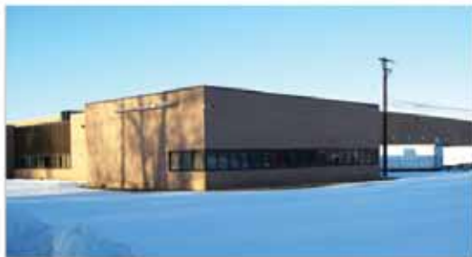
Warehouse Newark, New Jersey 250,000 sq.ft
