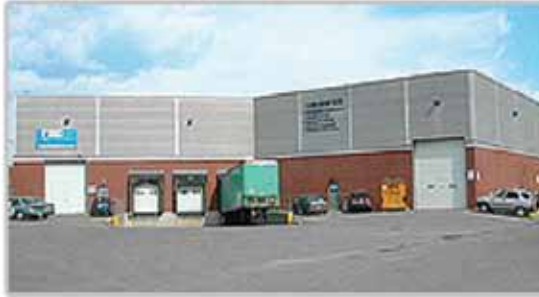
Warehouse Montreal, Quebec 71,000 sq.ft
